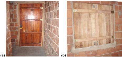
Figure 1: (a) Batten door used in PS1; (b) Window used in PS1
