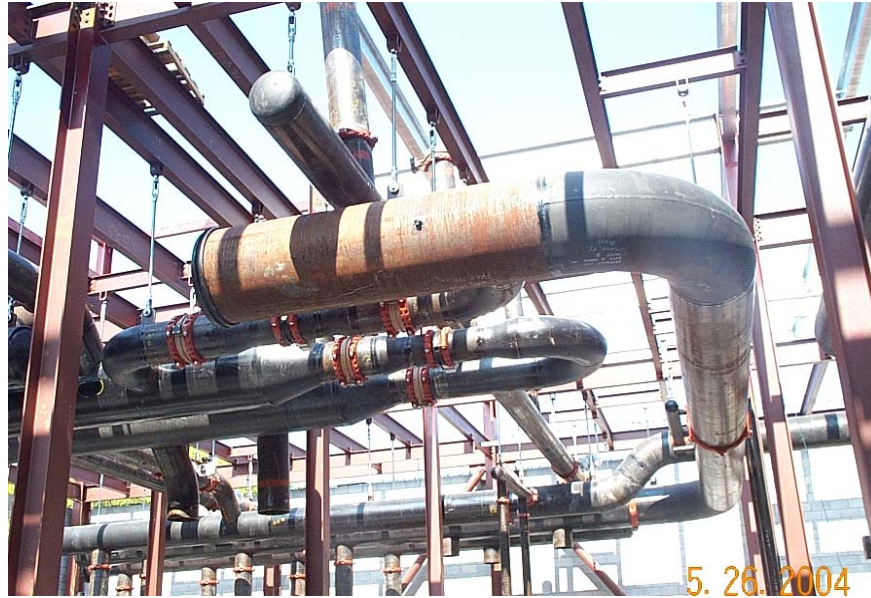
Figure 8. Pipe hoisting and installation using special crane.
