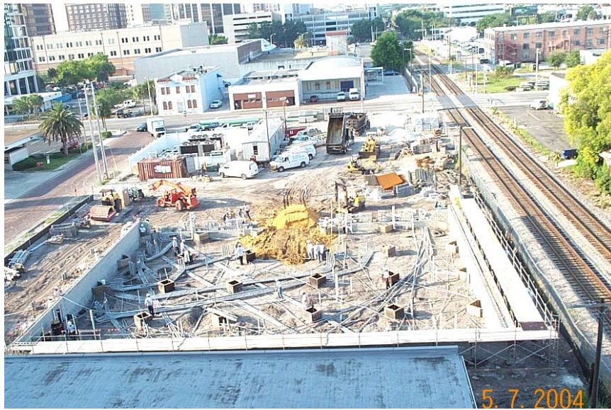
Figure 3. Installing under-slab utilities 5
