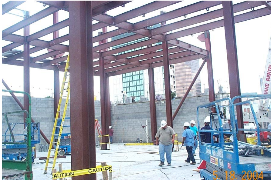
Figure 6. Structural steel beginning to take shape.
